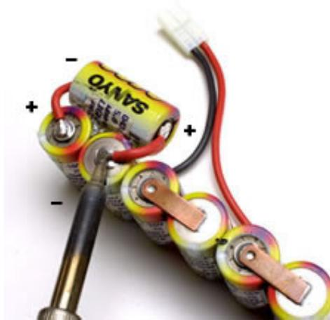
Then connect the negative terminal of the fifth cell to the positive terminal of the seventh cell and solder. Your pack is now complete.
