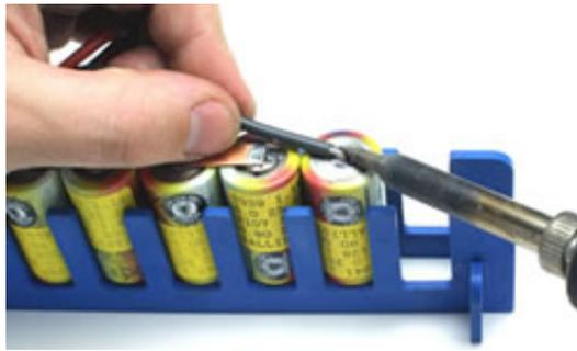
Solder the end of the red wire onto the positive terminal of the first battery and the black wire to the negative terminal of the sixth battery.
