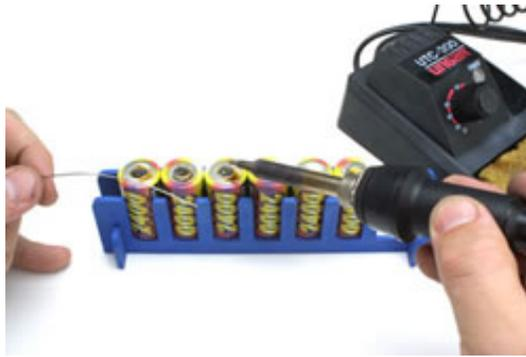
Do this with each cell. Now your cells are tinned. Now, tin the battery bars. Tin each end of the battery bars on one side (face).
